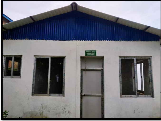
Waste management building Ilam Hospital
